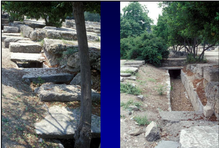
Stormwater drainage channels in the Agora, Athens, Greece, built by Peistratus in the 6 th century, BC and still working today.
